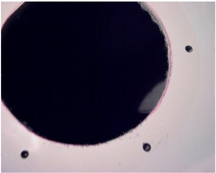
Using jigsaw, carefully cut out opening to 1/8" greater than marker line. Beckson recommends a loose fit (to be filled with silicone) to allow for heat/cold expansion.
